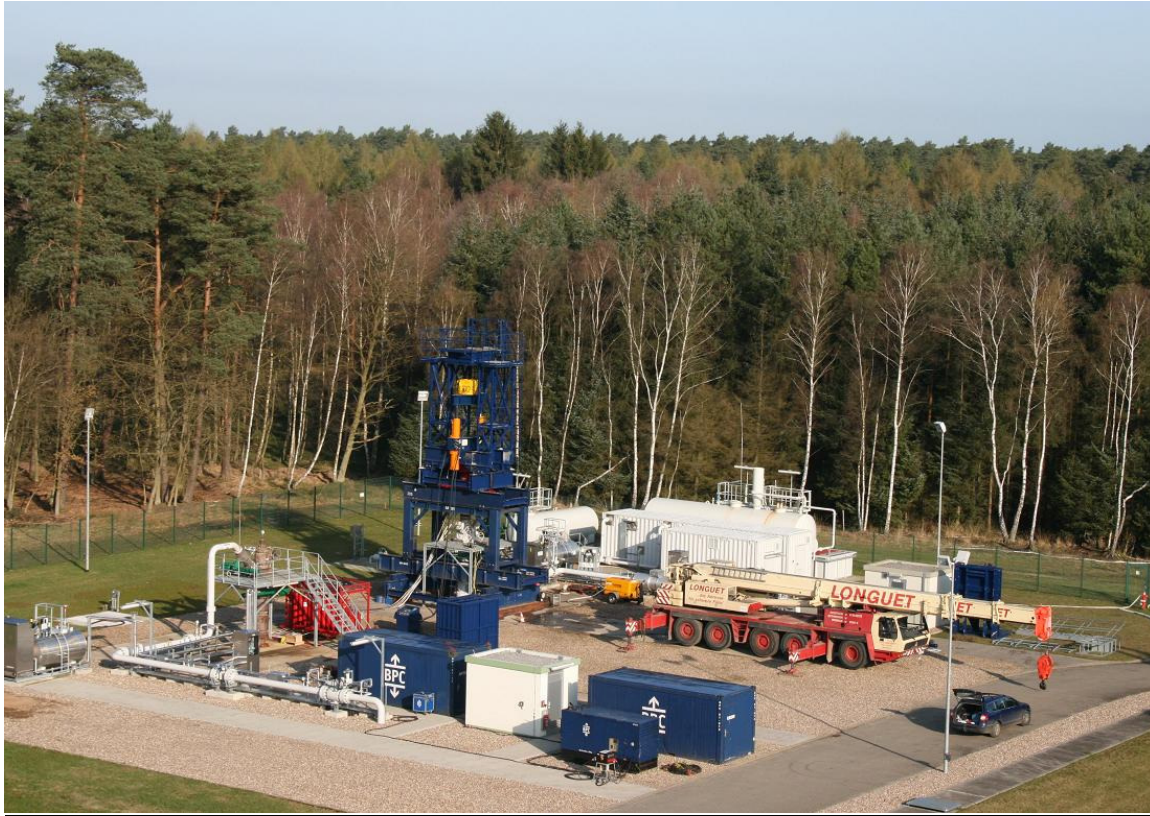
260T Pipe Pulling Unit on a location in Germany
