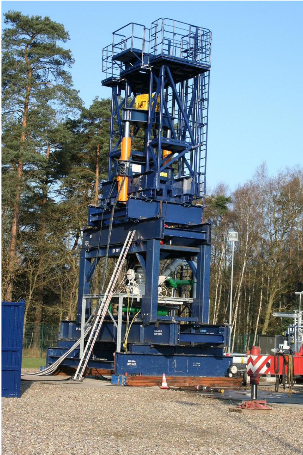
260T Pipe Pulling Unit
